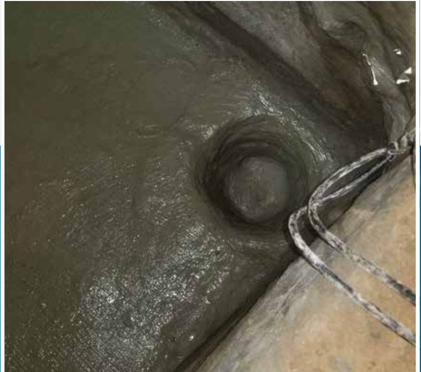
Old Rubble Foundation Elevator Pit Sealed, NYC.
