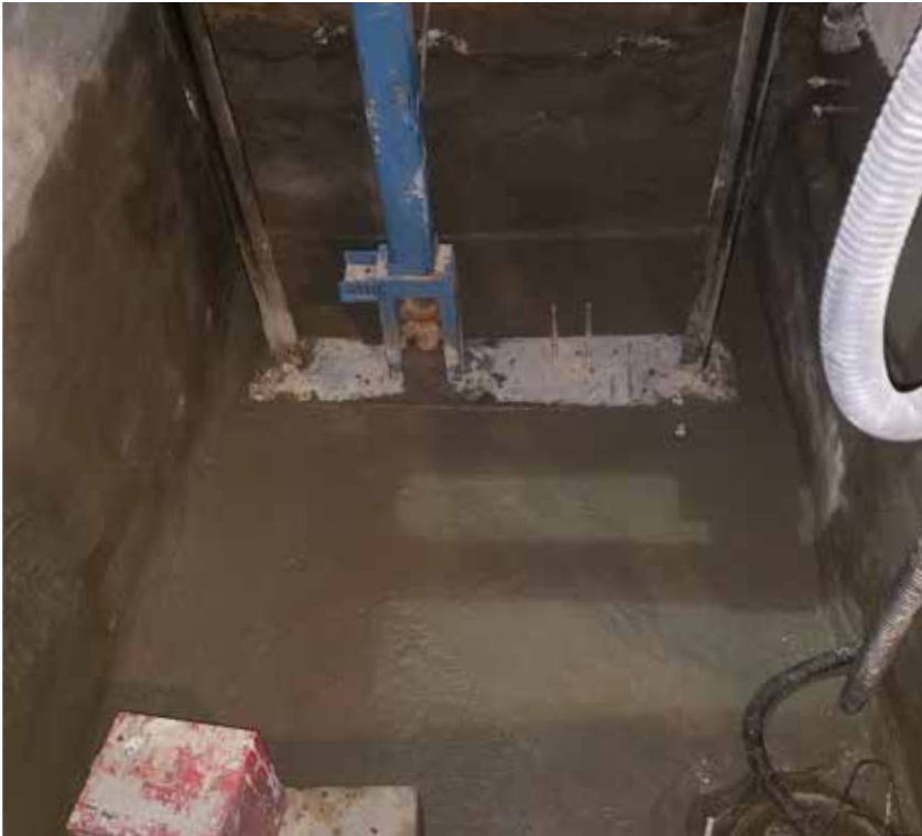
Elevator Pit in water table Sealed, NYC.
