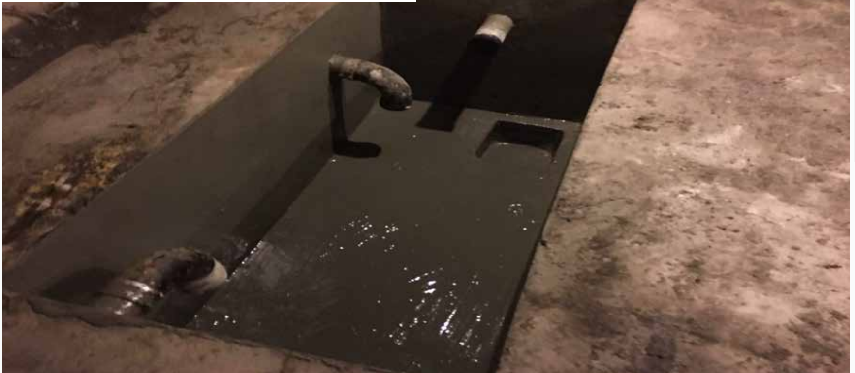
Ejector Pit In Water table sealed, Brooklyn NY
